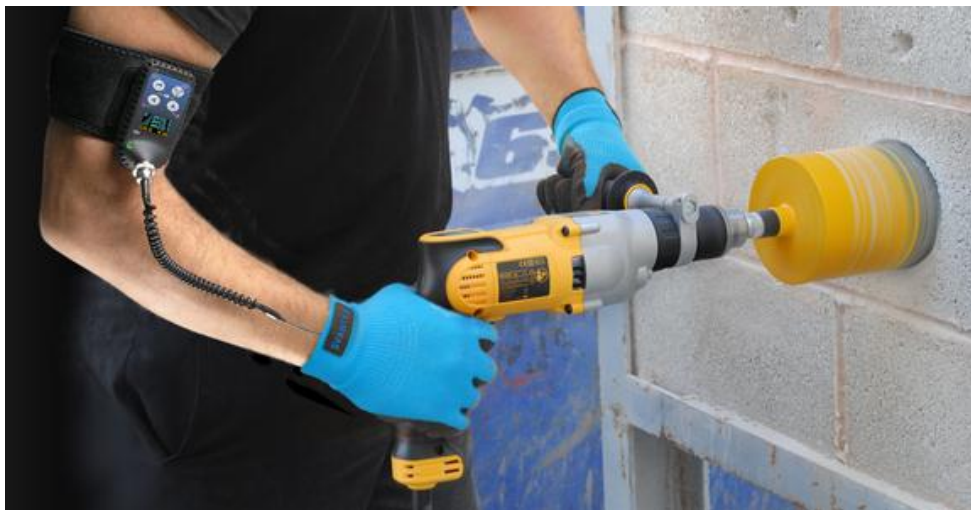
Photo 4 Typical mounting of SV 103 vibration exposure level meter on an operator's arm
